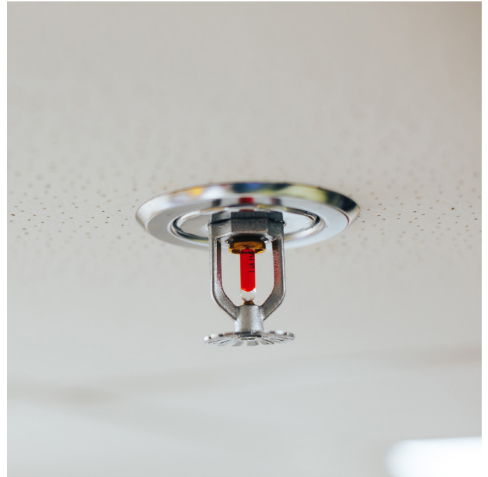
This image shows a clean, intact, appropriately positioned escutcheon plate.
